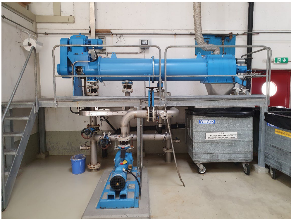
Figura 4 – Strainpress.
